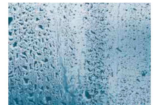
The glazing is tight from the inside of the room, therefore no humid room air can enter and damage the timber.
