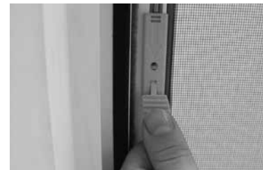
1. Open the window. Hold the friction fit frame on the plastic clips and put into the frame clearance on the outside. Position the bottom brackets first between the window frame and the gasket.
