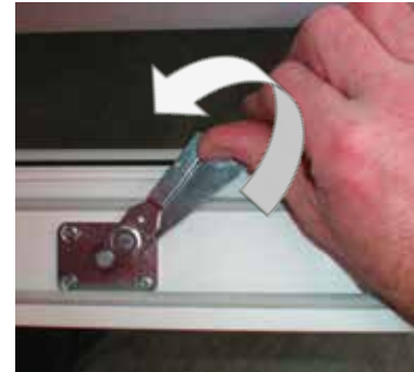
Open rebate stay-arm lock, unhinge rebate stay-arm and bring sash into cleaning position.
