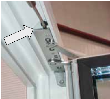
Adjust towards hinge or handle side with 4mm Allen key.
