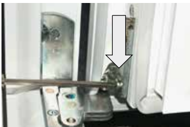
Adjust closing pressure with 4mm Allen key.
