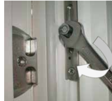
Adjust required contact pressure with fork wrench SW11. Adjustment is available in steps of 22.5°.
