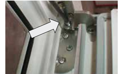
For heavy-duty hardware use torx T25.
