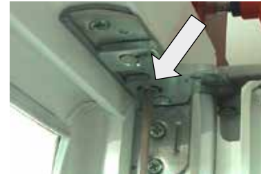
Adjust towards hinge or handle side with 4mm Allen key.
