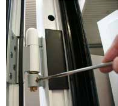
Loosen fixing screw.
