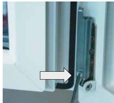
Adjustment of turn limiter with 2.5mm Allen key, if right-handed - with sash closed, if left-handed - with sash open.
