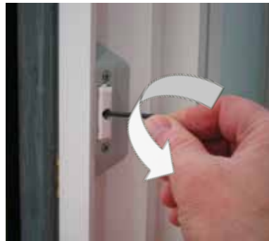
Adjust the catch with 3mm Allen key.
