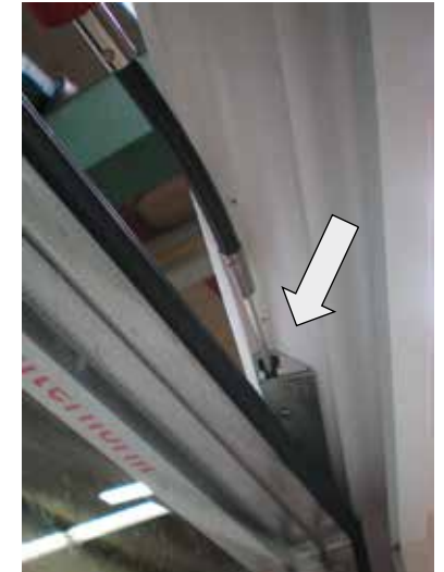
Raise and lower sash with 4mm Allen key.
