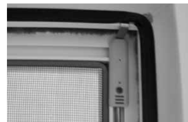
2. Pull the friction fit frame into the frame clearance so that the top brackets can also be positioned into the window frame by moving the plastic clip up. Afterwards fold the plastic clips down.
