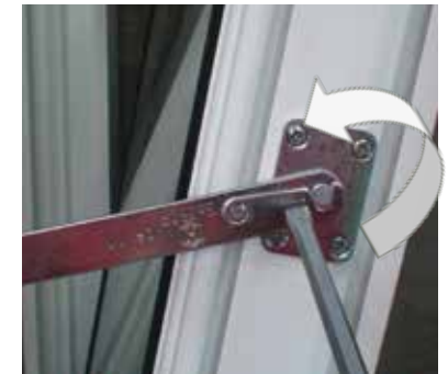
Open cleaning stay-arm lock with slot screw driver and unhinge cleaning stay-arm. Secure sash!!
